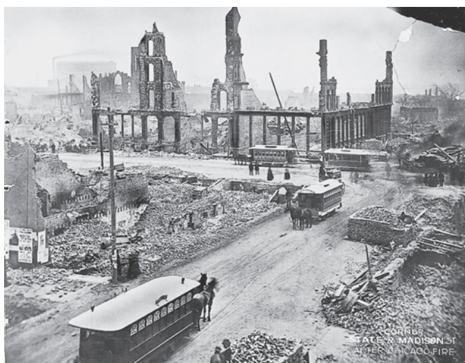
Aftermath of the fire of 1871
